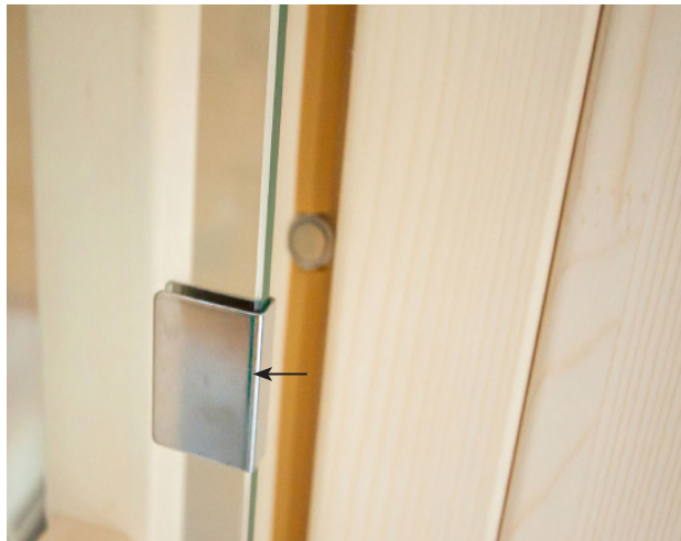
Fig. 35: Assembly of sleeve plate
