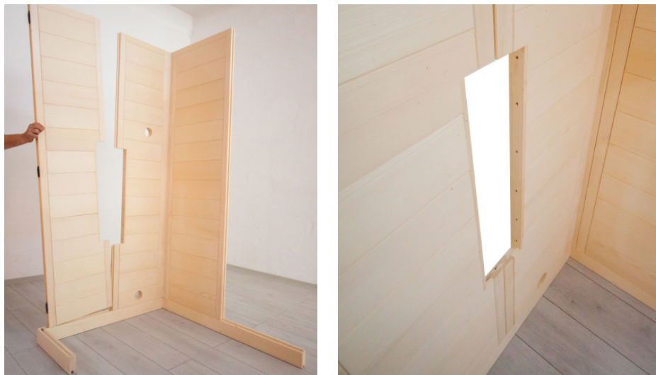
Fig. 6: Inserting wall element with recess
