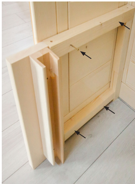
Fig. 18: Installing the bench supports
