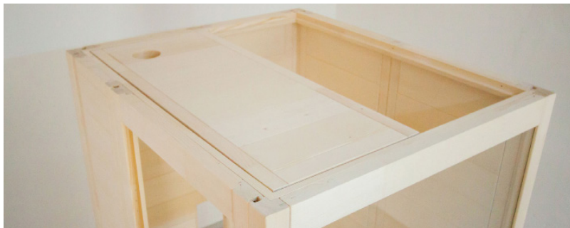
Fig. 14: Inserting front ceiling element
