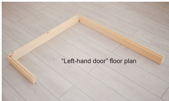
Fig. 1: Laying the three base frame elements
