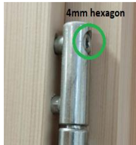
Fig.2 Frame horizontal direction adjustment bolt
